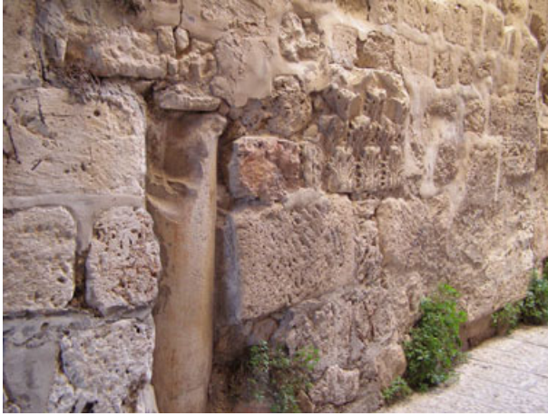
FIGURE 1. “Spolia”— A Roman column inlaid in a sixteenth century wall, the Old City of Jerusalem.
